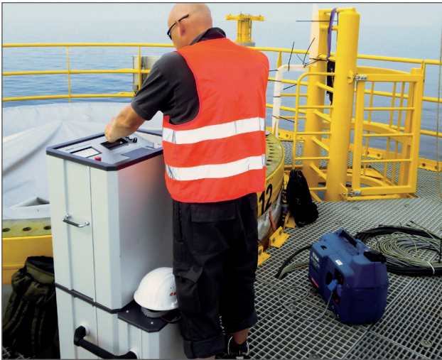
VLF CR-60 kV in operation on the "Baltic 1" wind park (Baltic sea).
